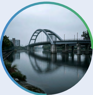
Bay, river, and lake crossings
