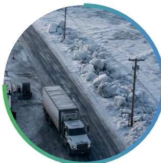
Temporary winter roads and ice road installations
