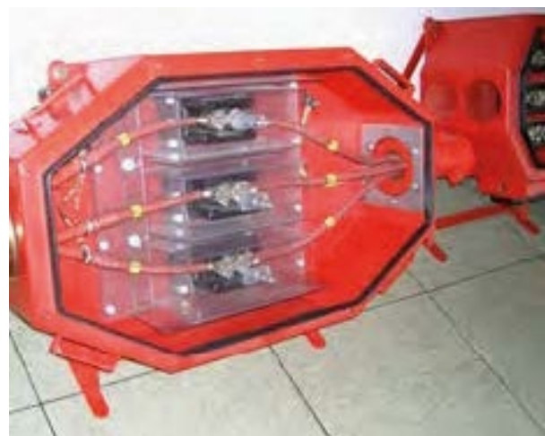
Special sealing end termination for connection box.
