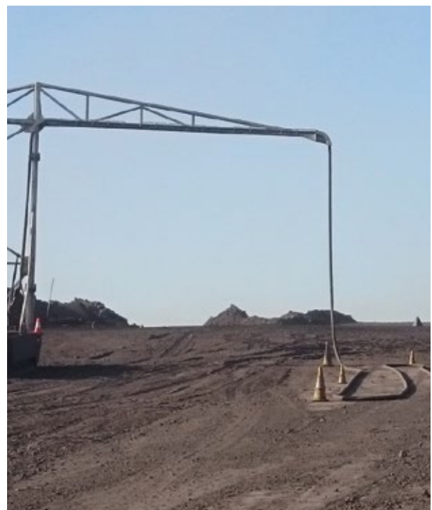
Cable suspended above guideways
